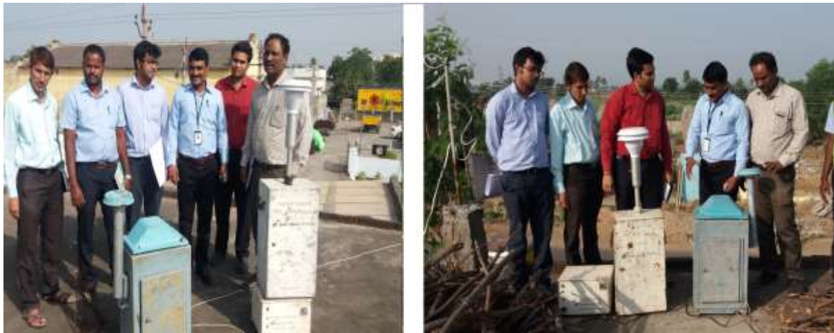
Figure 6-7 AAQ Monitoring stations installed at Malkapuram and Velgapudi
