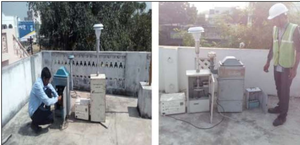
Figure 6-13 : AAQ Monitoring stations installed at Dondapadu and Navuluru
